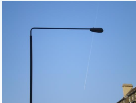
Street lighting – $2,656 each new or $664 for an upgrade
